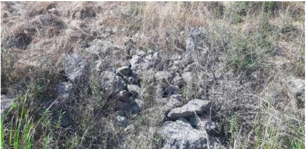
Photograph 5 : Dislocated rock pieces on the downstream slope of ash pond 2
